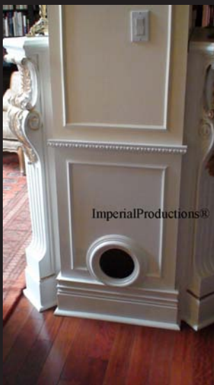
Cut out as Air Return
