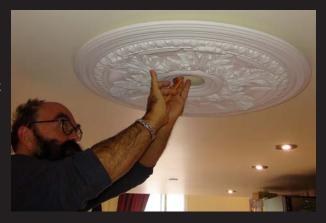
7) Apply the Adhesive. Use approved adhesive only that is safe for ArchPolymer<sub>TM</sub> - put multiple small blobs on the back side of the medallion. Use this same adhesive for Neo-Plaster-GRG
