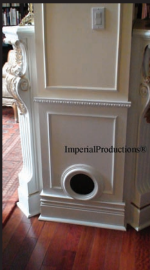
Cut out as Air Return
