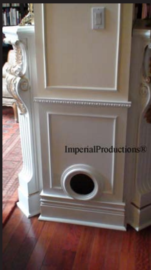
Cut out as Air Return
